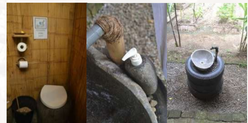
Figure 3. Toilet and Sink
